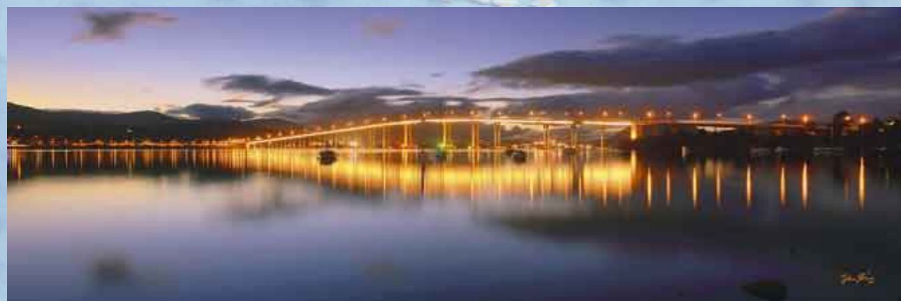
P145 Tasman Bridge - Hobart, TAS, Australia
